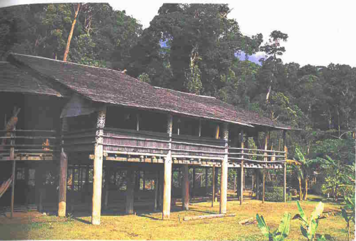
Front view of Orang Ulu longhouse. The projecting verandah denotes the beadman's quarters.
